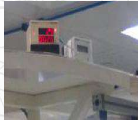
Precise Temp Controller Interfaced to HVAC Blower Motor
