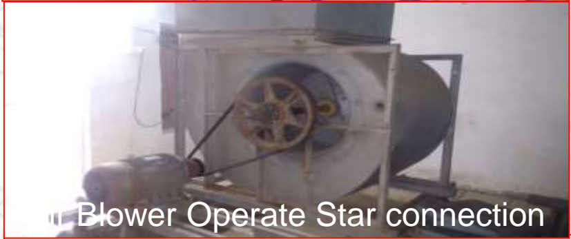
Star Connection in AHU panel
