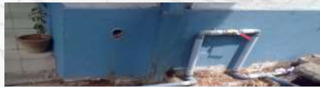
Under Ground pipe line Removed above the ground Valve ½ Position used
